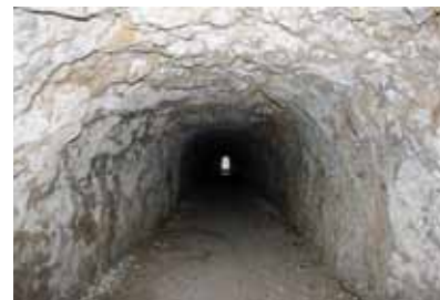
Dynamite, which has nitroglycerine as its active component, can be used to blast tunnels through solid rock.
